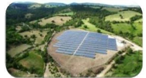
PROJECT YEAR: 2016 CITY: ÇANAKKALE 4,235 MW
