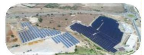
PROJECT YEAR: 2017 CITY: AYDIN 5,5 MW
